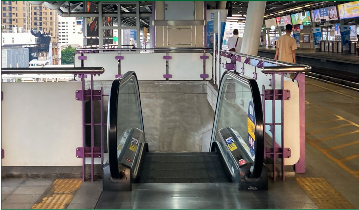
Guard Area between Escalator Rails and Rail Wall Panels.
