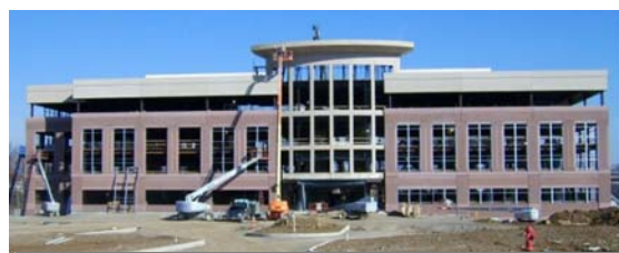
Safety National's new headquarters under construction
